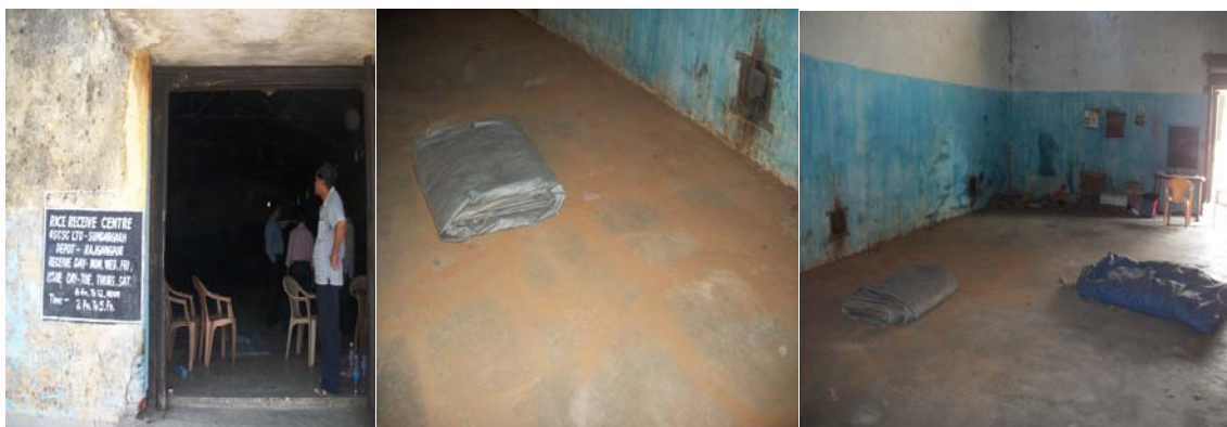
RRC at Sundargarh in wretched condition
